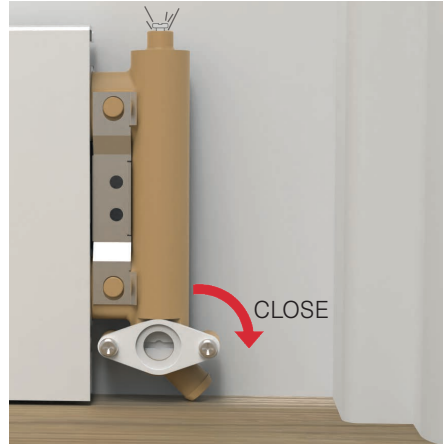
Return Manifold BM2: Clockwise Installation
