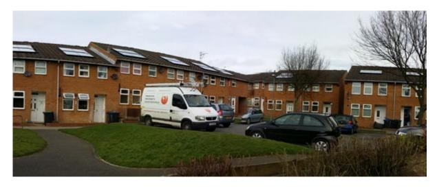
A typical ThermaTwin system will deliver between 900~1,000 kwH per year, typically sufficient to provide 60~70% of a 2/3 bed properties annual hot water requirements
