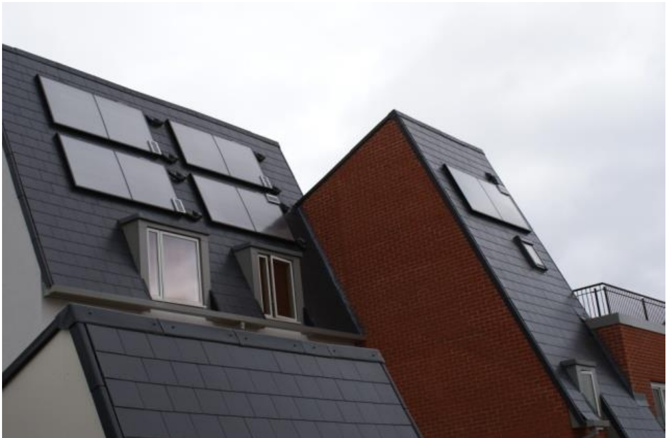
Over 200 ThermaTwin panels have been installed in the Village
