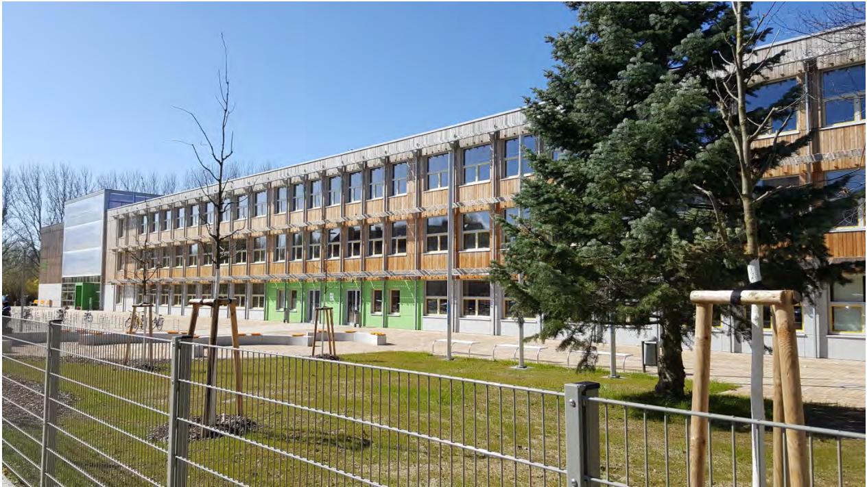
Rostock Energy Plus School produces more energy than it consumes
